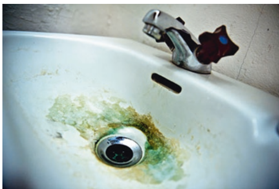
Fig. 4.2 Green precipitates of copper from copper pipes in a public sauna, Värmdö, Sweden (Frejning 2012)
