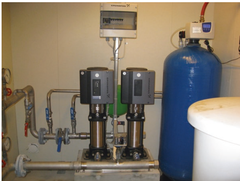
Fig. 6.6 Softener, ion-exchange filter, in a residential community in Sweden (Photo: I Rosborg)
